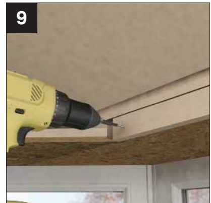
9 Attach additional mating timber battens.
