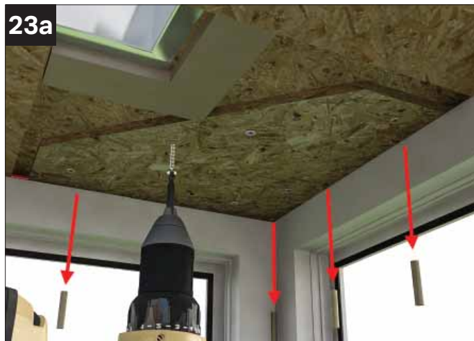
23a Remove timber positioning dowels (see step 3b). Fix up through the front 90° beam support shelves into the box beam using 6x5.0 x 50mm countersunk wood screw (RRX 025) provided. See fixing points at 22b (standard soffit) and 22c (extended soffit).
