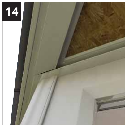
14 External ship lap cladding edge channel detail.
