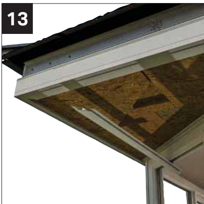
13 Fit external ship lap cladding edge channel.
