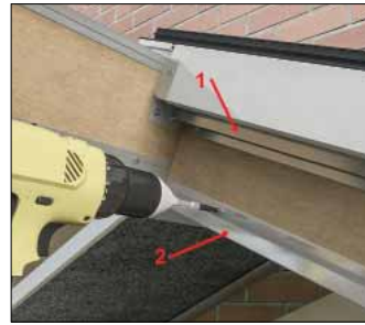
Refitting lower channel 'U' number 2
