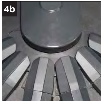
4b On 3 and 5 facet victorians after tiling, fit the preformed external tile flashing trim (NRVT001). Secure into position using 2 x screws (NRTS 050) provided.
