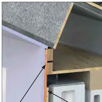
Additional 12mm OSB cladding on internal Loggia face (supplied) Existing external loggia OSB cladding
