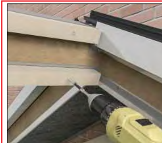
Fitting of the timber ridge battens
