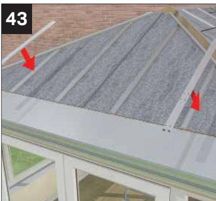
When all panels installed continue to fit the pre drilled external panel clips (see next image for positioning alignment)
