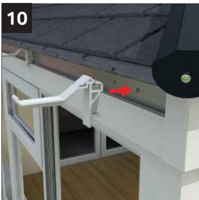
10 Fit gutter bracket by placing lower leg onto aluminium gutter channel then 'snap back' upper leg. Space at maximum 750mm centres and within 200mm of corner.
