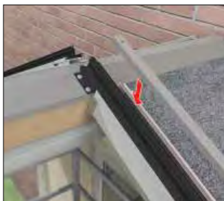
Fixing glazing bar to ridge
