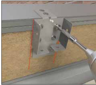
Fixing glazing bar shoes to ridge section
