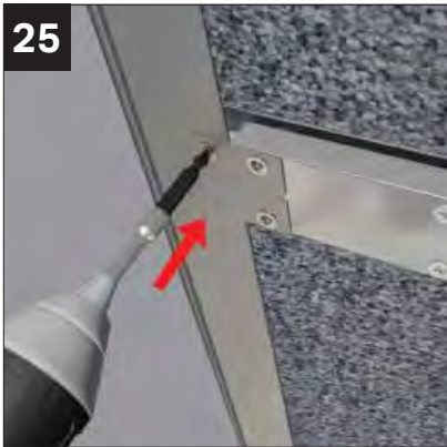
Secure to the ridge body, the upper attachment plate using 4 x NRTS 050 fixings.
