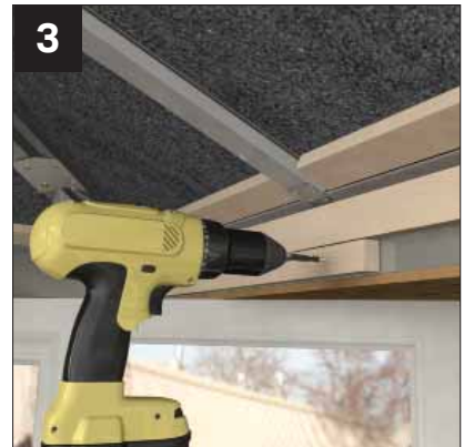
3 Attach additional battens.
