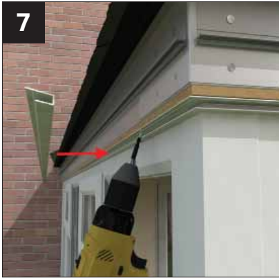
7 Screw fix PVCu soffit channel into head of window frame or base of OSB board (screws not provided).
