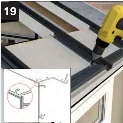
Secure the glazing support section at 200mm ctrs using NRTS050 4.2 X 25mm screws provided.
