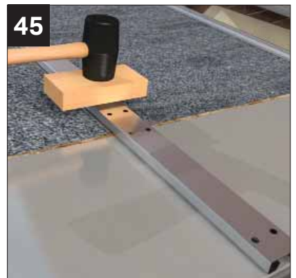
When aligned use a robust mallet to knock down the external panel locking clips (use a short length of timber to protect the clip from indentations).
