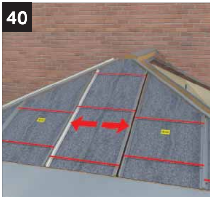
The expandable panel will expand to take up any tolerance gap. Snip the binding cord on all the remaining front facet panels.
