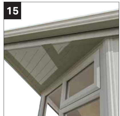
15 Cut and fit ship lap to suit.
