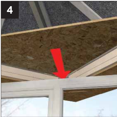
4 Slide into position additional external OSB board.
