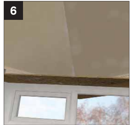
6 Plasterboard the roof.
