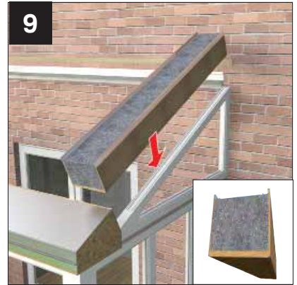
Locate end panel (s) onto the rear wall plate shelf and box beam shelf. Ensure OSB boarding on end of gable panels are flush with the end of the beam. Note: if there is glazing against a return wall see page 25. Marked with a yellow label, all gable end panels are supplied with OSB (timber panels) to the inside face.
