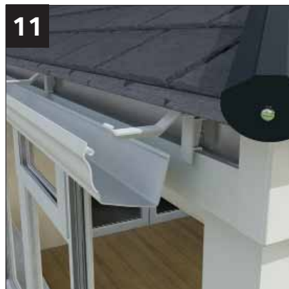
11 Fit Marley Classic guttering. Ensure when fitting the gutter you fit to the insertion marked lines within the unions / gutter corners.
