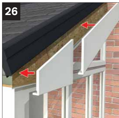
26 Fit the pre-cut fascia and eaves trims. See page 50, images 26 to 29 for more detail.
