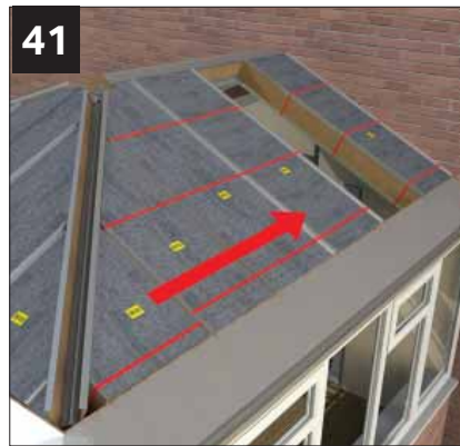
Repeat the process on the side facets.
