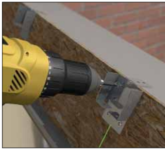
Fixing glazing bar shoes at box beam
