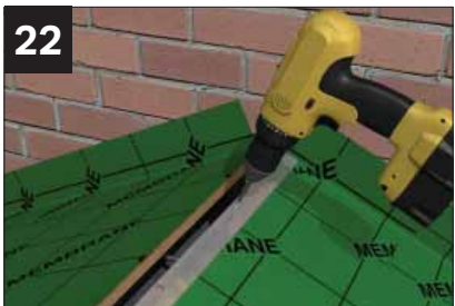
At each side of the glazing area, an aluminium upper tile stop is fitted. The lower edge of the tile stop is positioned a set distance from the edge of the bottom tile starter support. See critical dimension sheet for dimension A, see step 29. The tile stop is bedded down with clear low modulus silicone, then screwed at 300mm ctrs using (NRSF012) 4.8 x 38 pan head screws provided. Finally seal lower edge of the tile stop to underlayer again using clear low modulus silicone.
