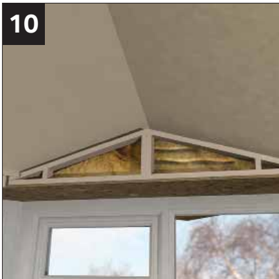
10 Insulate void with mineral wool.
