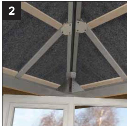
2 Batten out to suit plasterboard fixing.
