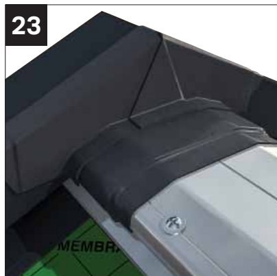
23 Finally cover joint with a third layer.
