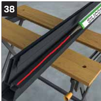
Apply a bead of clear low modulus silicone to the underside of the dry verge.
