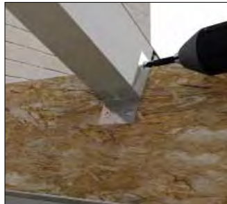
Fixing glazing bar at box beam shoe
