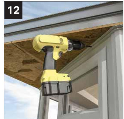
12 Fit external soffit channeling.
