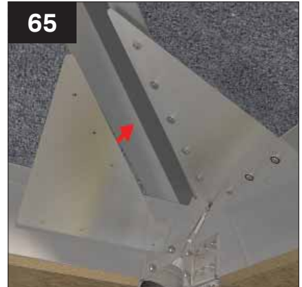
65 Fix the internal hip retaining plates using 18 x CHAA 006 screws provided.
