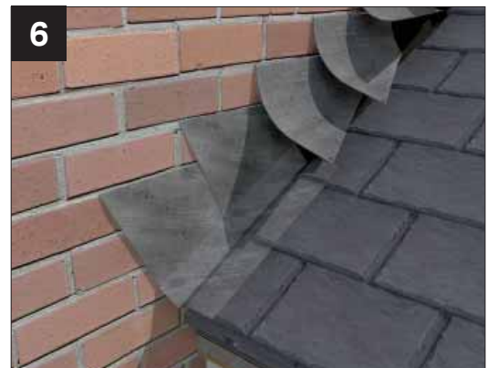
6 If using existing flashing, dress down over the roof and ridge area then finish as normal. Flashing may need trimming to fit neatly. Apply patination oil to lead for peace of mind (Avoids unsightly lead sulphate run off). Alternatively install new code 4 lead.
