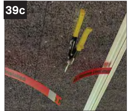
When in position snip the retaining straps.
