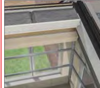
Fitting upper plasterboard trim
