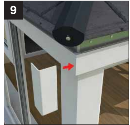
9 Fit PVCu fascia corners with silicone.
