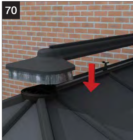
70 Offer up the complete ridge capping onto the roof.
