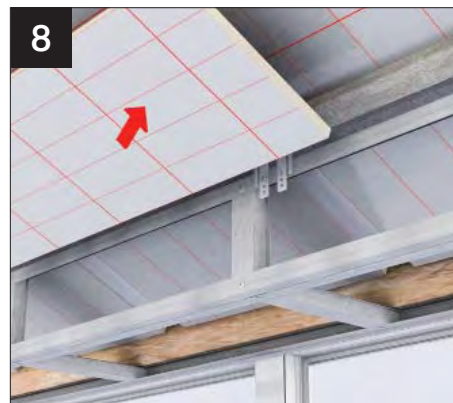
8 Next fit the 25mm insulation board, which is 590 x 2400mm. These boards must be laid at right angles to the glazing bars and run across the bars.
