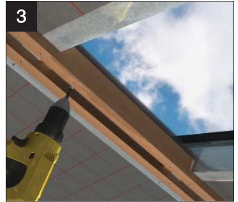
3 IMPORTANT: POSITION CLOAKING PANEL ASSEMBLY 6MM BACK FROM THE CROSS BATTEN (AS SHOWN) SCREW FIT INTO POSITION.
