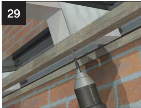
Fit additional battens where glazing is present along the host wall as shown.
