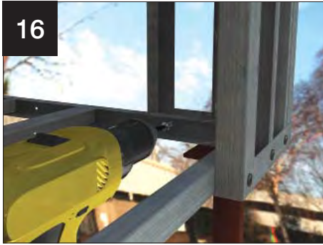
Fit the valley corner infill panel to the horizontal frame, level up and secure to the valley plate.
