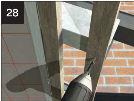
Fit second row of battens as described on page 40.
