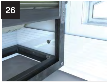
26 Fix the vertical frame into the fascia board using 2 x CHA006 (M4 x 13mm) self drill Phillips, wafer head screws (supplied).
