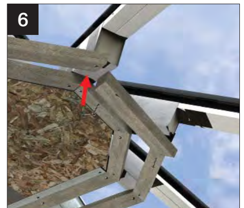
6 Using drywall screws, attach battens into steel bolsters/stub steel bolsters.
