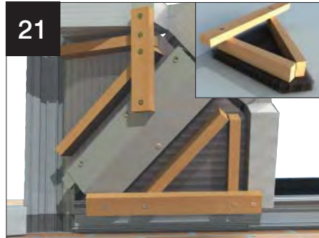
Fit modesty panels adjacent to valley – create cassette assembly as shown using double sided tape to fix battens to the polycarbonate and screw fix the support batten into position as shown. Offer up the modesty panel into position to define the position of the support battens.
