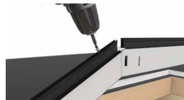
2 Secure the bell rafter using the pre-fitted retention screw.
